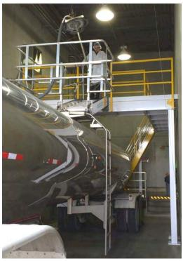
A custom engineered mezzanine was contracted and installed with a drop down stairway with integrated protective fall cage for tanker hatch access, allowing safe operations and ease of training new personnel. Total cost Approx. \$24,000.
