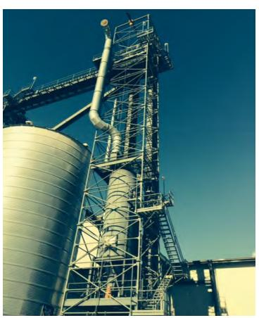
A hoist was installed so that heavy equipment can be easily hoisted up. Now team members have their hands free to use handrails while climbing the steep stairs.
